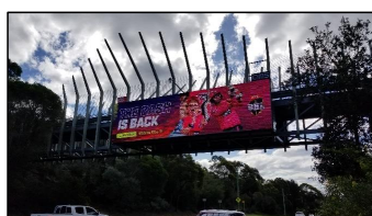
Figure 14. Exterior view of the west side of the pedestrian footbridge. Taken from the south side of Wentworth Avenue, facing east.
