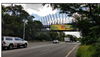
Figure 15. Exterior view of the west side of the pedestrian footbridge and Wentworth Avenue below. Taken from the south side of Wentworth Avenue, facing east.
